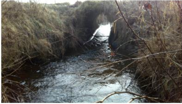
Station 2040 rørbro Ø 120 cm set opstrøms
